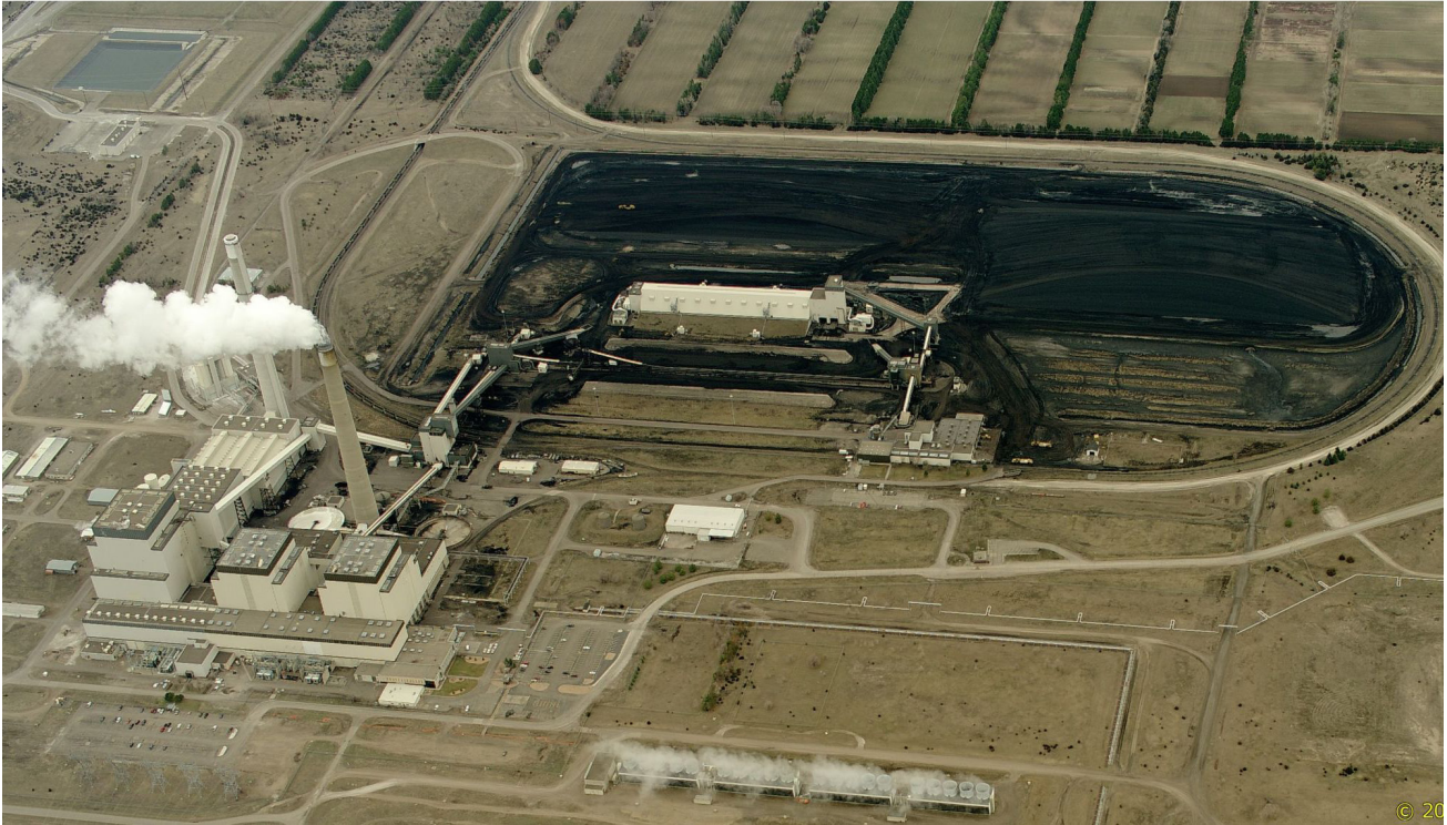
Becker, MN - Example of industrial (energy coal) of rail user
