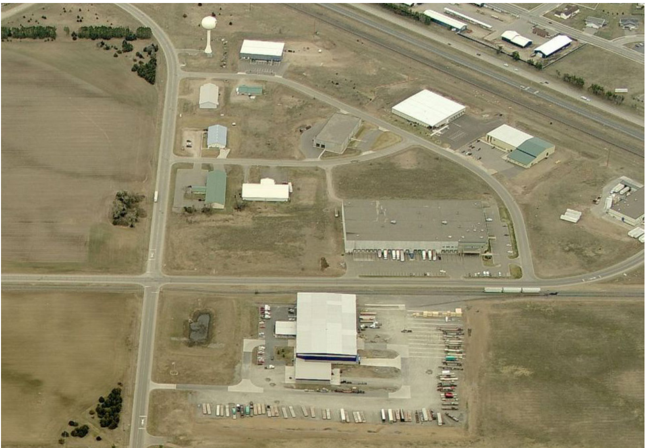
Becker, MN - Example of light industrial/manufacturing rail user
