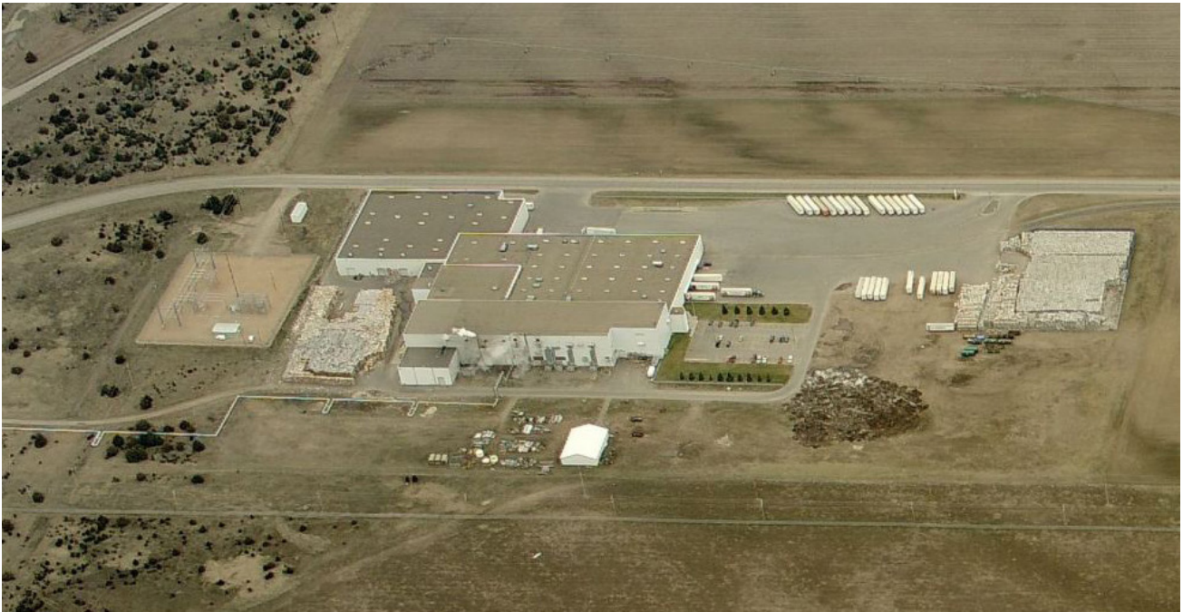
Becker, MN - Example of light industrial/manufacturing rail user
