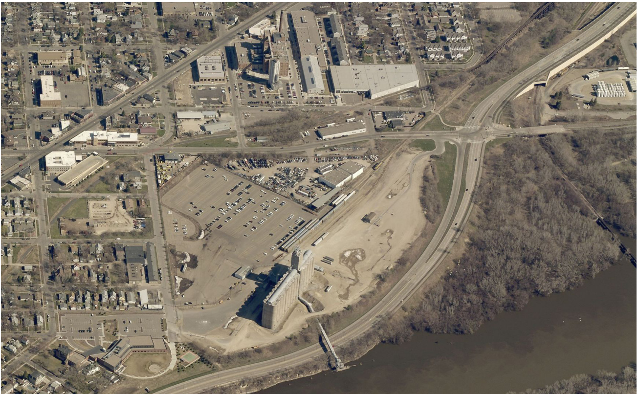
Saint Paul, MN - Example of transload facility (agriculture/urban) and transload/distribution of rail user
