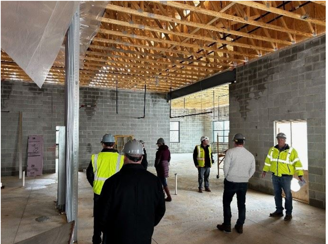
Figure 5 Truck bays in the maintenance building and office areas
