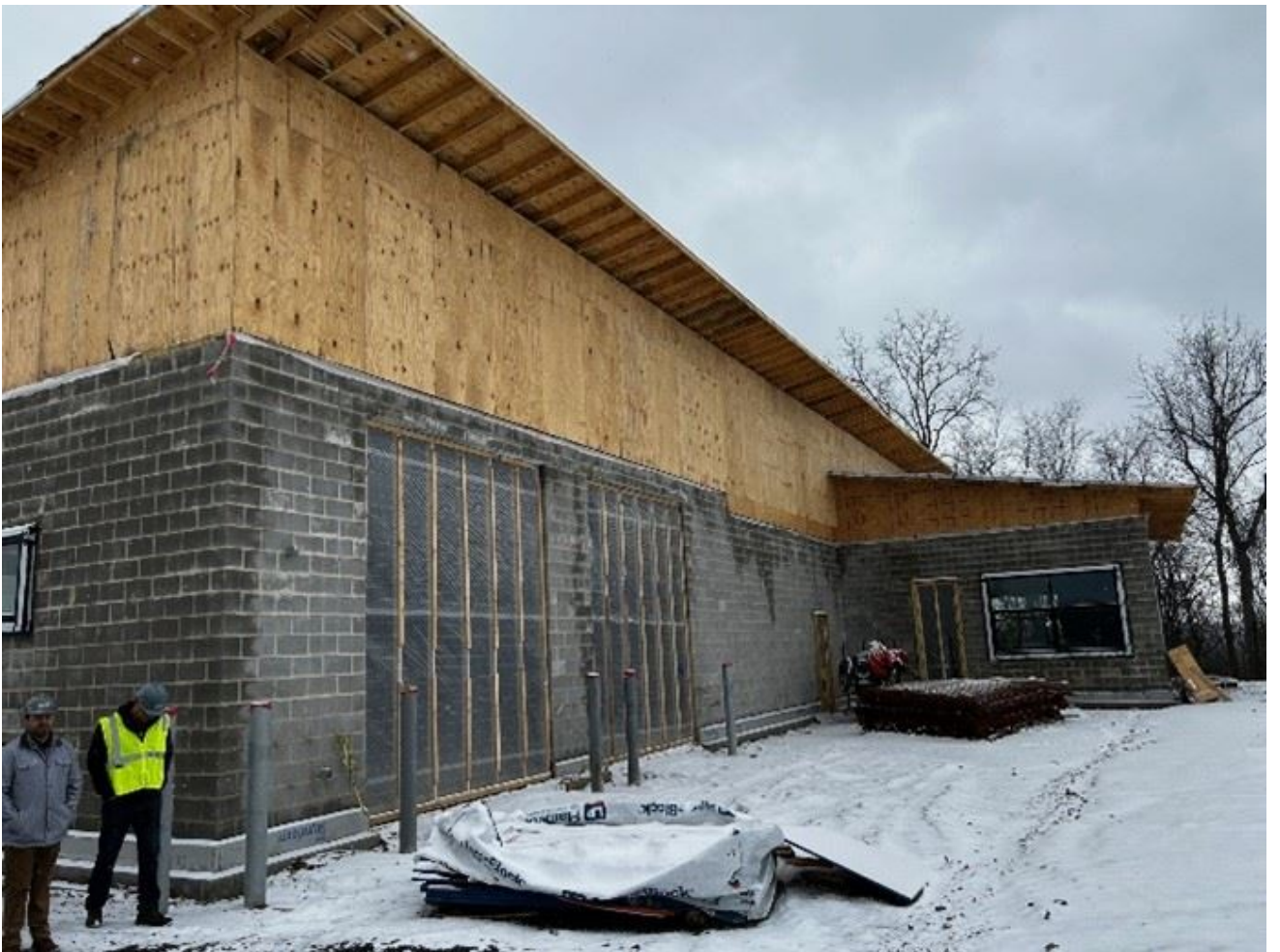
Figure 3 View of the walking path area maintenance building
