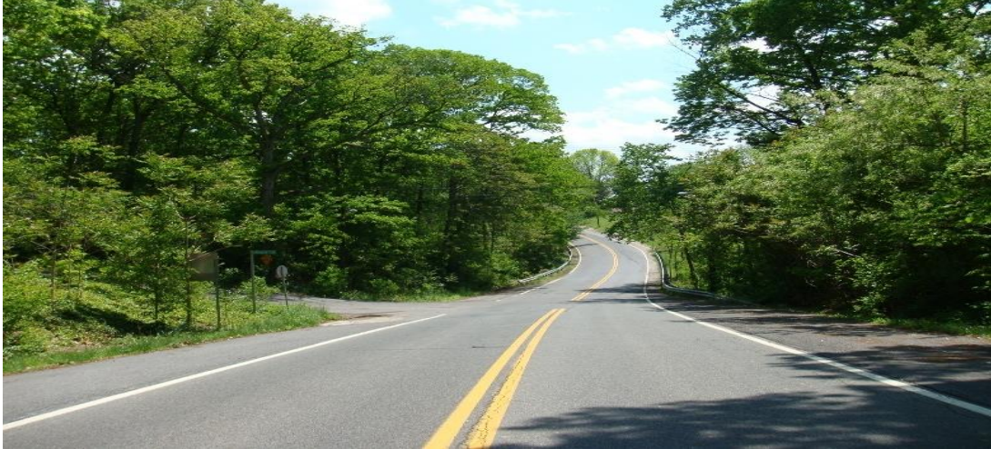
Figure 16: Transition from wide paved shoulder to narrow shoulder on Brooklyn Bridge Road.
