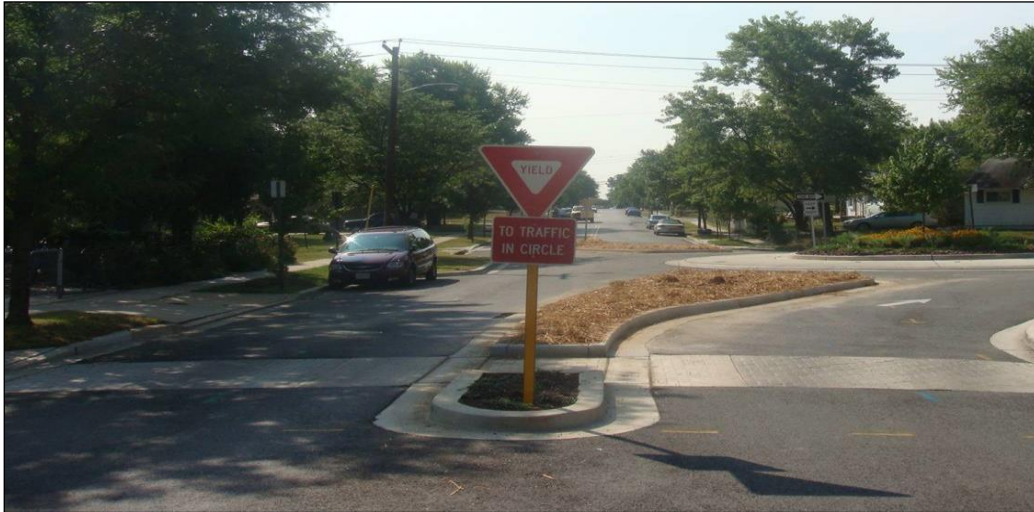
Figure 10: Traffic Circle at Intersection of Montrose Ave and Harrison Dr.
