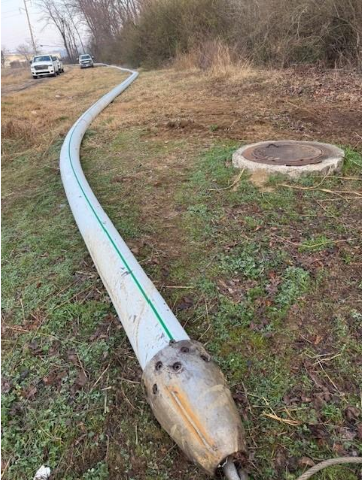
Fused HDPE Connected to Bursting Head
