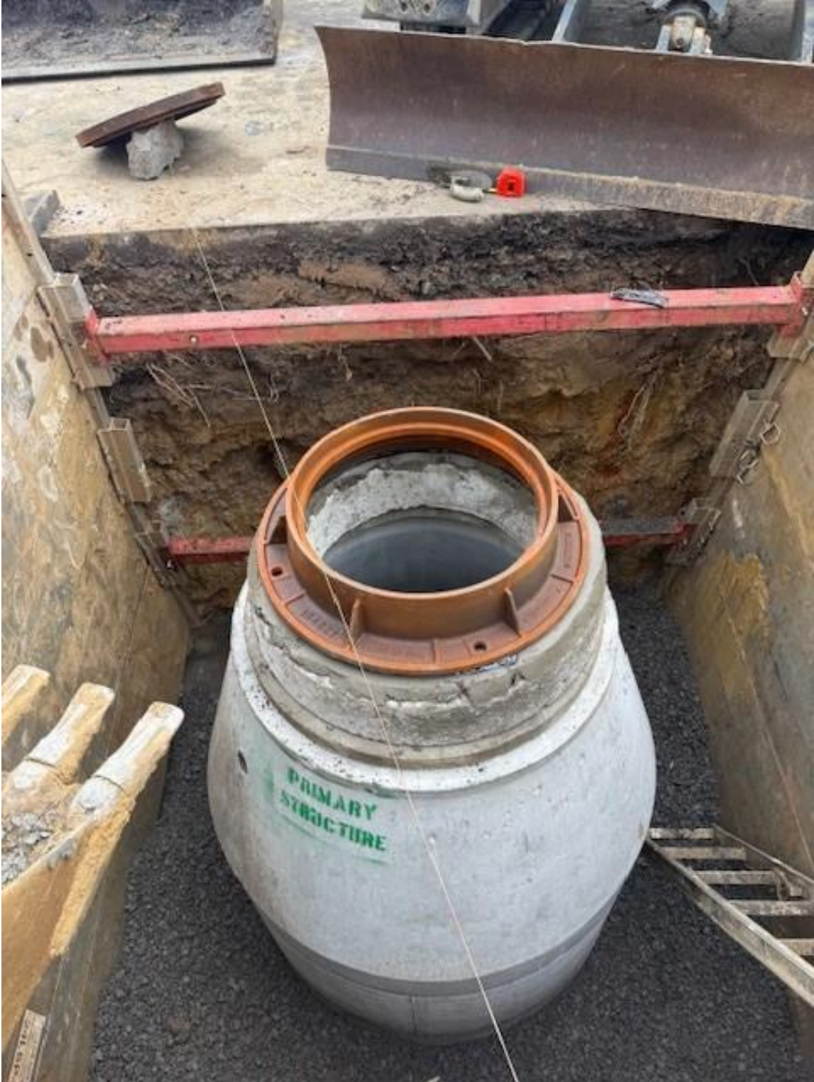
New 4-foot Precast Manhole with Casting
