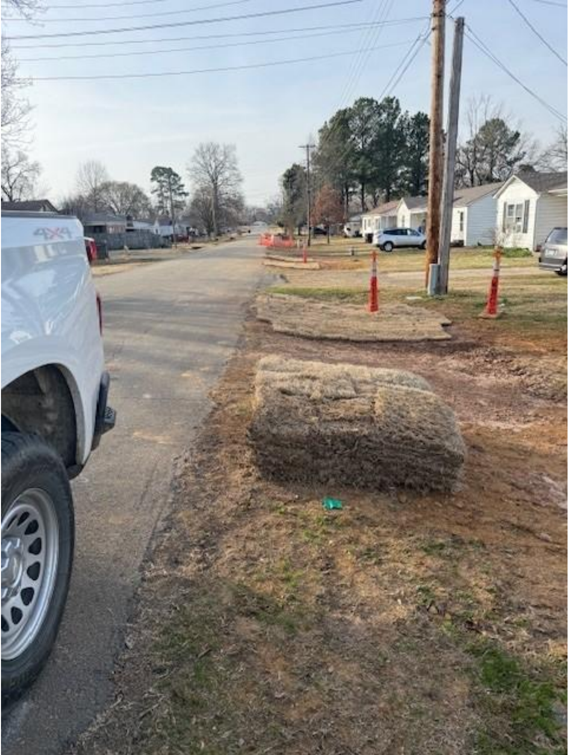
New Site Restoration Sod
