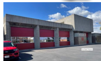
Overhead doors at Station #1
