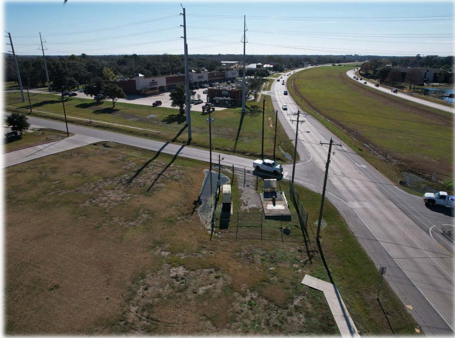
WWTP – Lift Station
