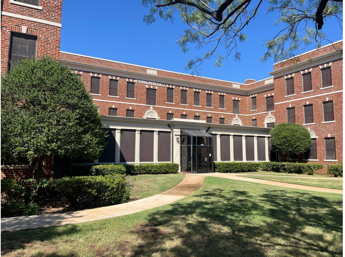
Photo 2. View of 1953 “lounge” addition on primary (east) elevation, view northwest.
