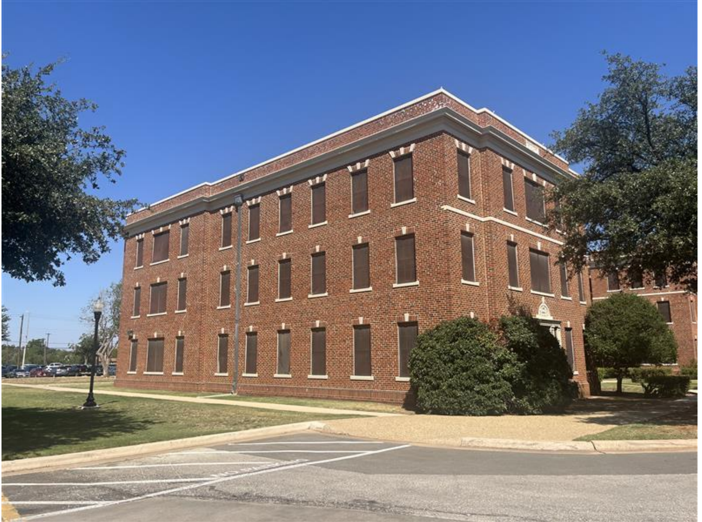
Photo 4. South elevation, view northwest.
