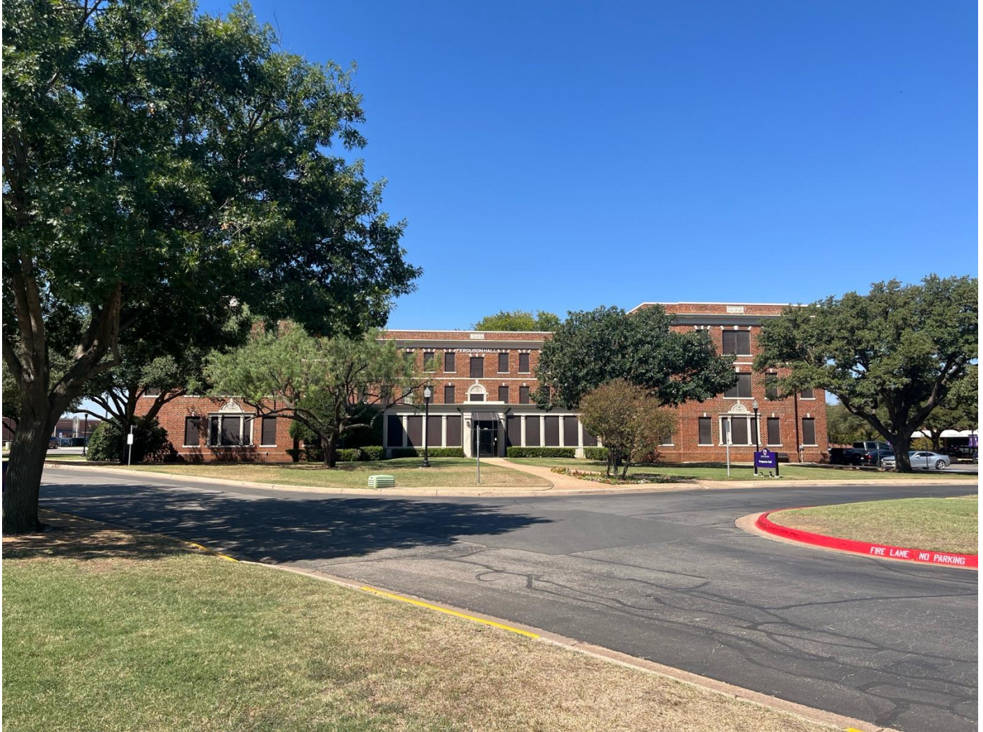
Photo 1. Primary (east) elevation. View west.
