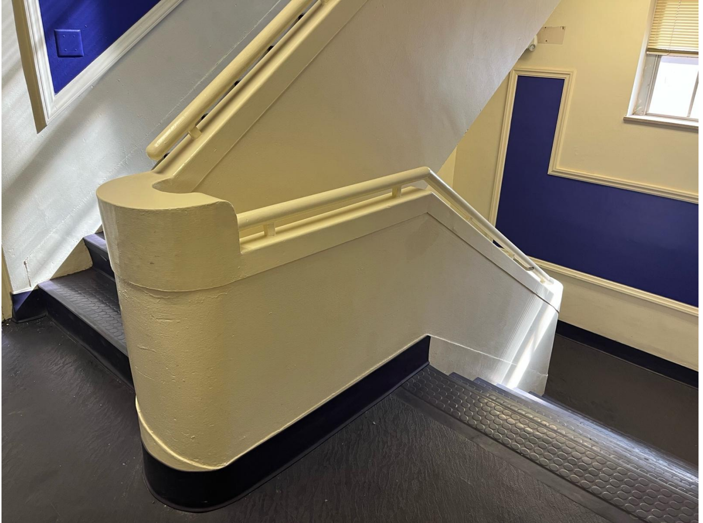
Photo 11. Stairwell detail, view northeast.
