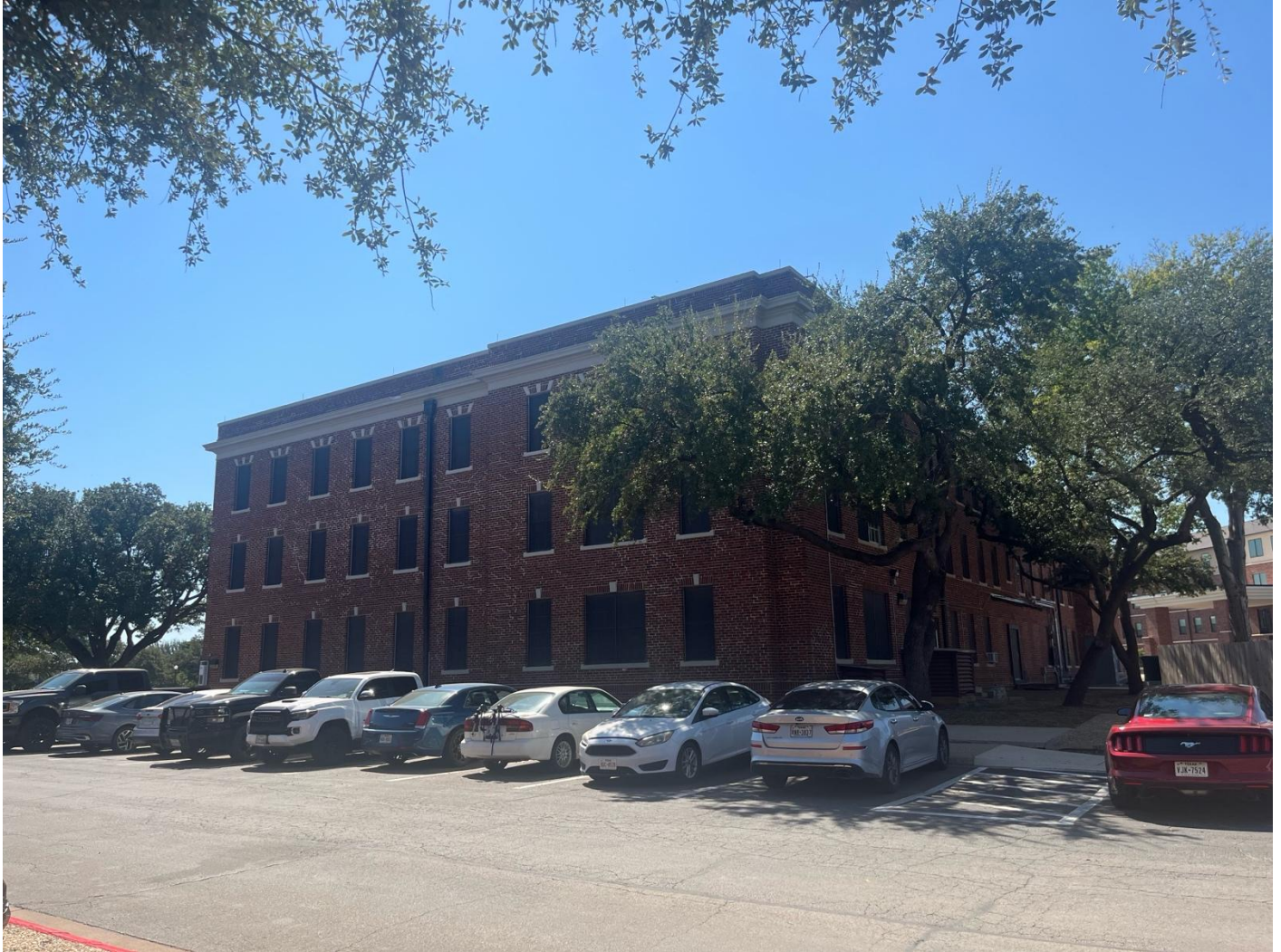
Photo 3. North elevation, view southeast.
