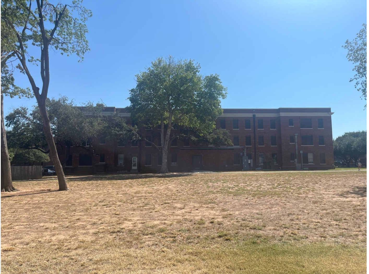
Photo 5. Rear (west) elevation, view east.
