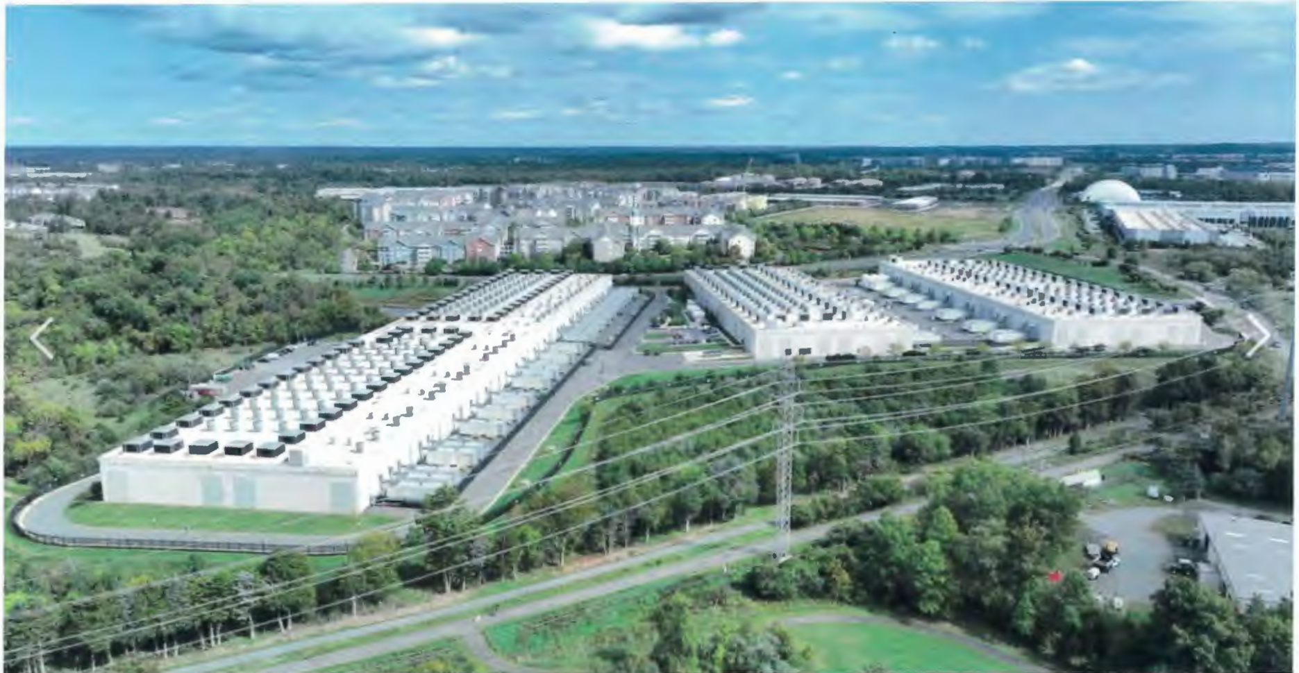
Microsoft's Gainesville Data Center (planned) 2,982 MW
