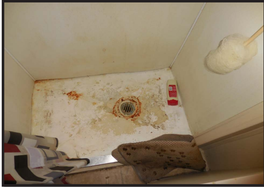
Rust in shower and mold on mat (Budget Inn, Broadalbin, Fulton County DSS)
