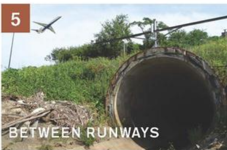
5 BETWEEN RUNWAYS The river appears briefly between culverts, below the elevated runways. The airport uses this opening to capture stormwater overflow and manage spills when they occur.
